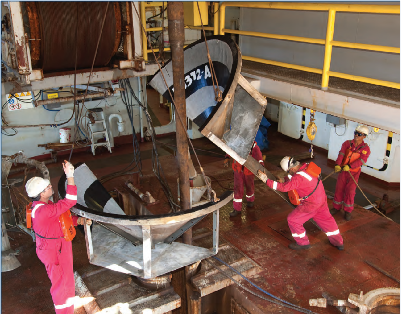
Assembling the free-fall funnel
