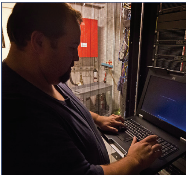
Checking the servers in the IT office
